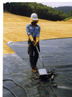
Joining the seam of a synthetic liner
